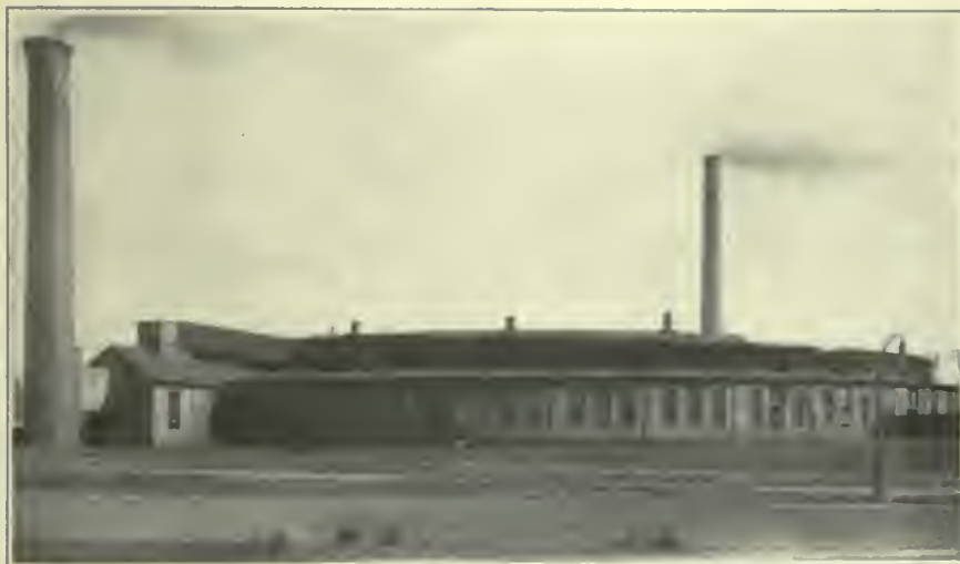
FIG. 351. LOCOMOTIVE TERMINALS. Engine House of the Chicago, Milwaukee & St. Paul Railway at the Western Avenue Yard.
